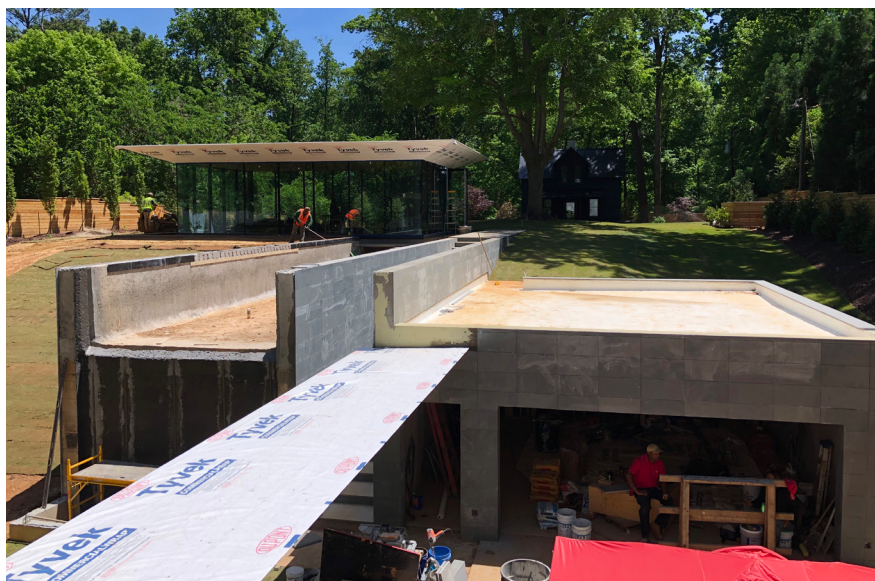
Fig 2 – Pavilion (background), pool and garage addition under construction. [photo courtesy Sheila Lee Davies]
